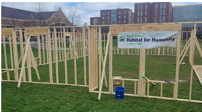
Building the exterior walls with the Habitat for Humanity Purdue Chapter on the Purdue University campus on April 21 for the upcoming Women Build.
